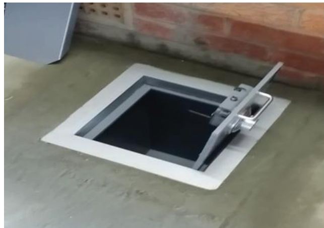
Figure 3 - Final Concrete Encasement
