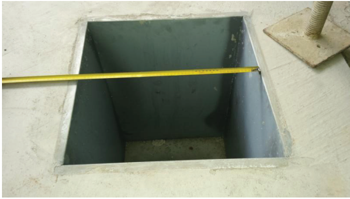
Figure 1 - Shroud set in the slab
